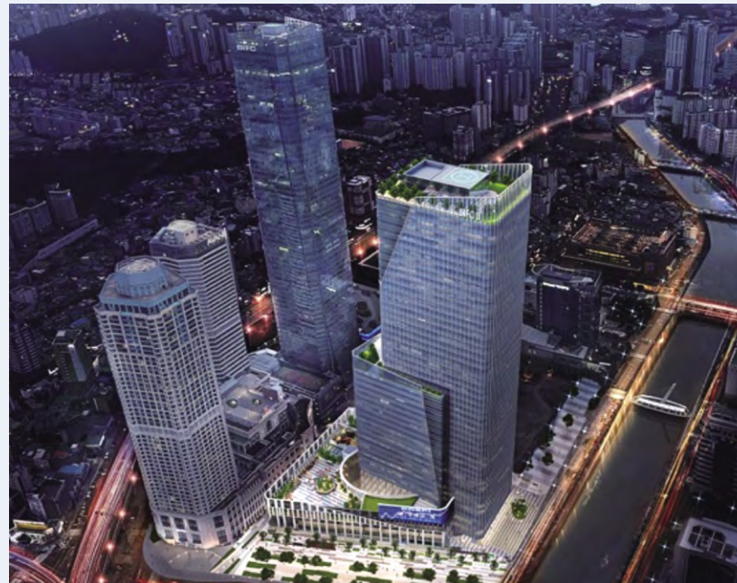
Busan BIFC phase 3 development project
